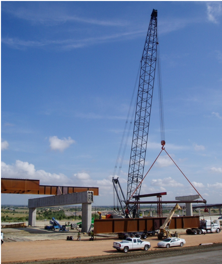
Figure 6.6 Crane Lifting Curved I-Girder
