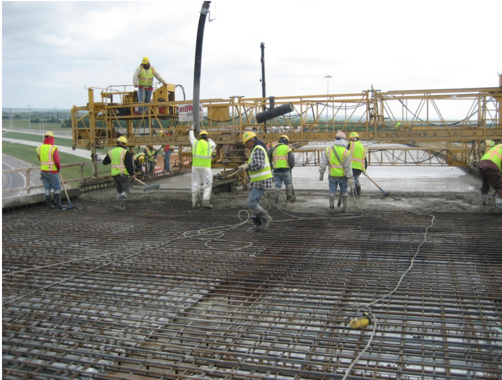
Figure 4.3 Transverse Screed used in deck construction
