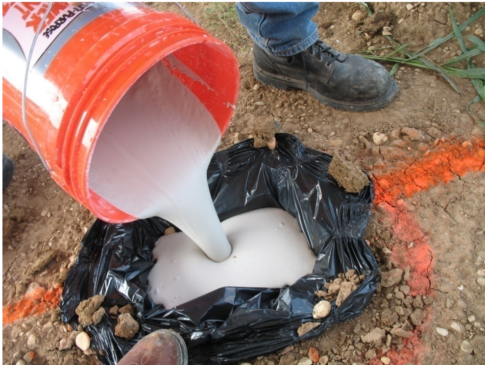
Figure 3.20 Pouring Hydro-Stone into hole
