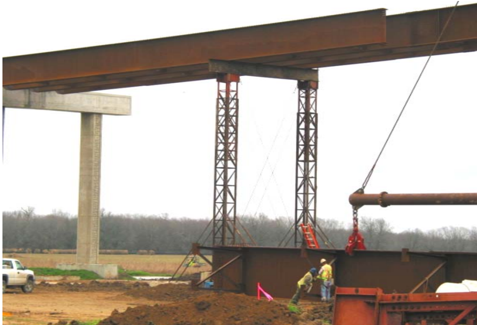
Figure 6.2 Shore Tower Supporting Curved Girders
