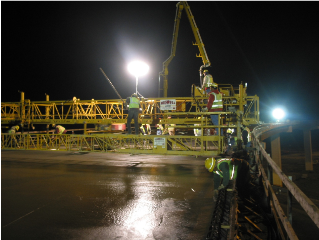
Figure 4.2 Concrete Deck Placement at beginning of pour
