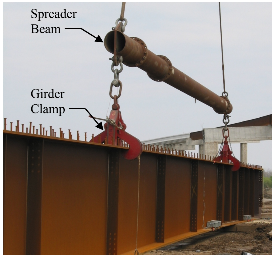
Figure 6.5 Spreader Beam Connected to I-Girder
