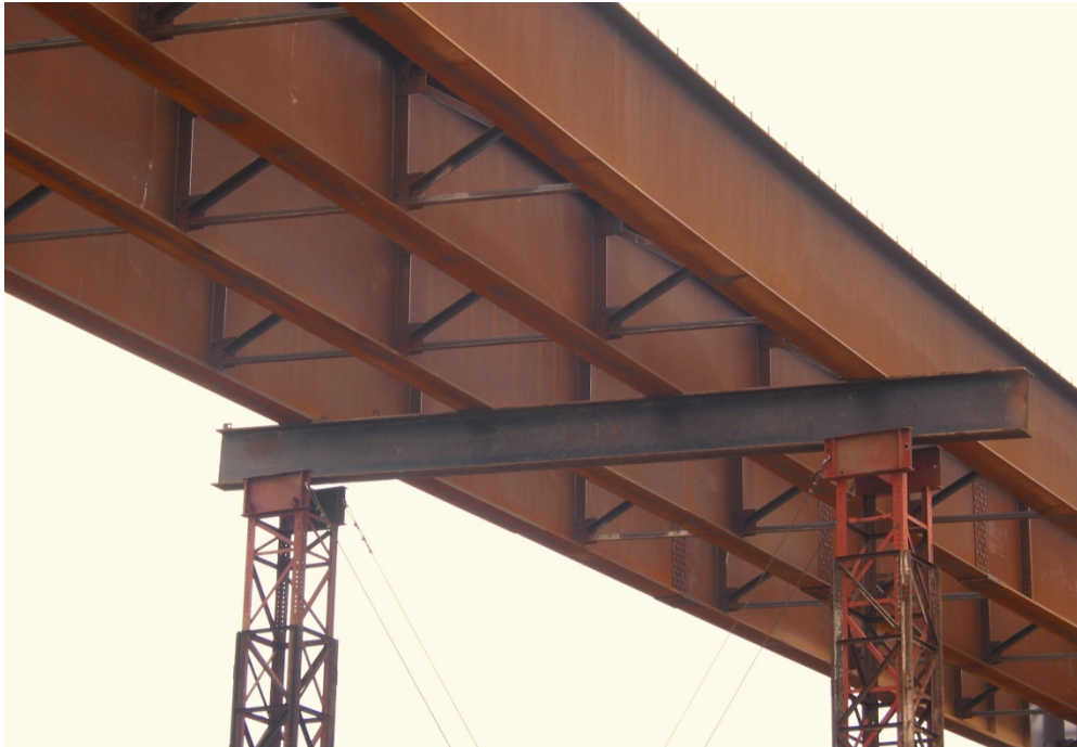
Figure 6.3 Shore Tower Beam Supporting I-Girders
