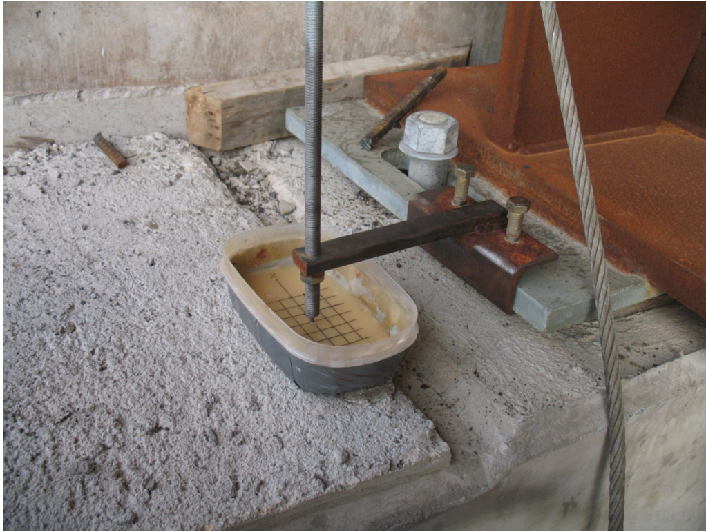
Figure 4.40 Wax Device attached to Bent 14
