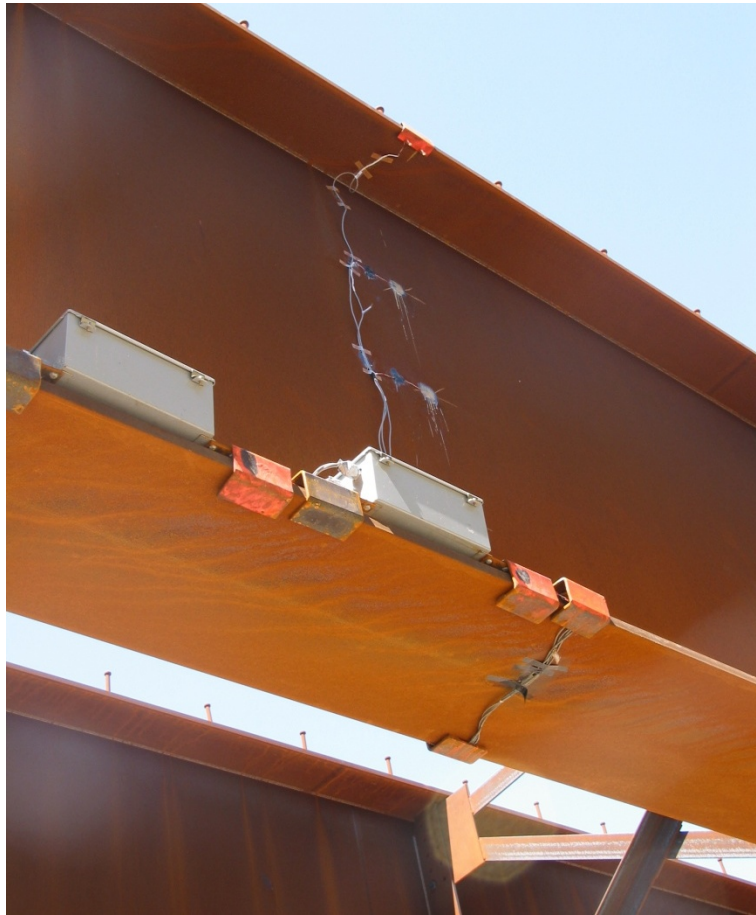
Figure 3.9 Dataloggers and Multiplexers protected in steel boxes on erected girder
