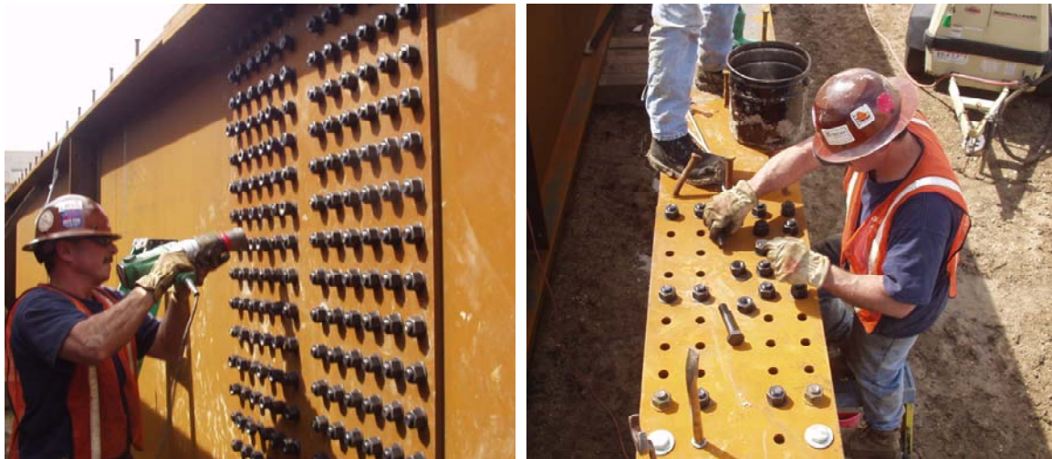
Figure 6.4 Ground Spliced Curved I-Girders
