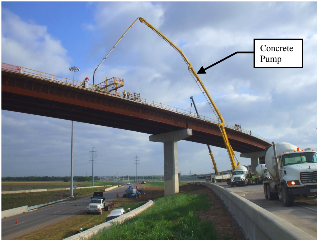
Figure 4.1 Bridge 88 Unit 3 Concrete Deck Placement
