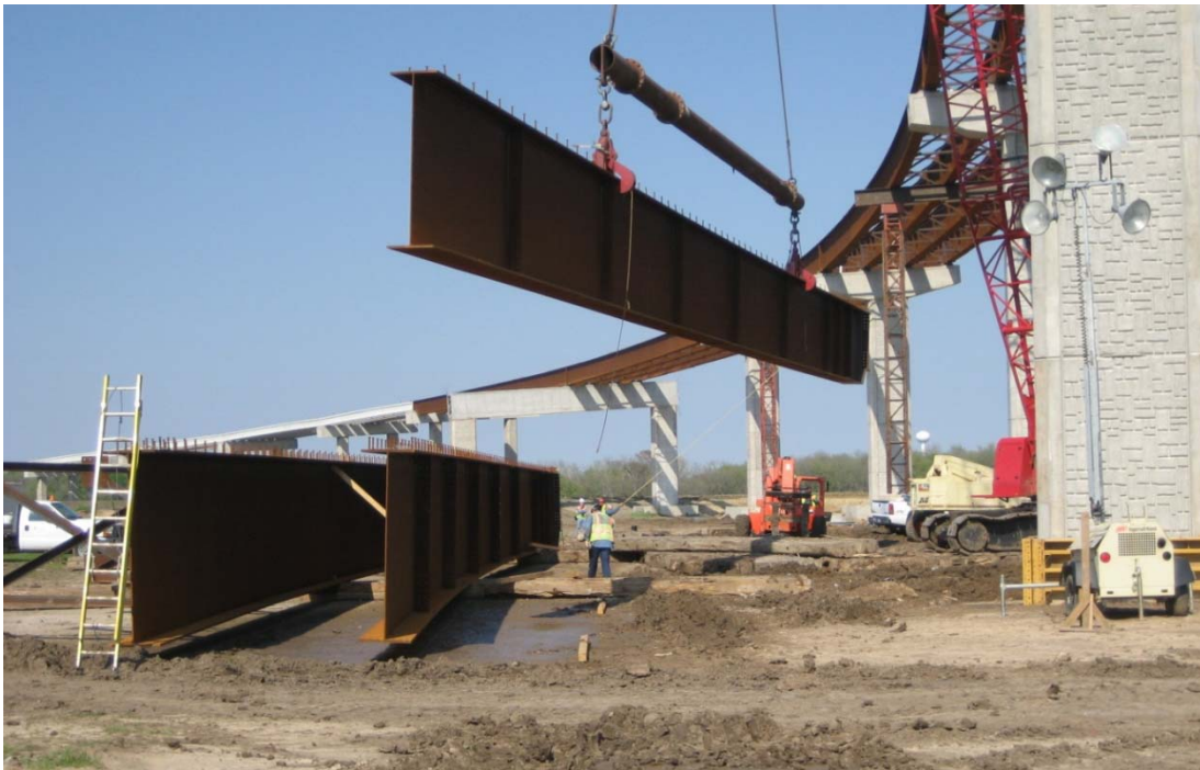
Figure 6.9 Lifting Curved I-Girder Segment
