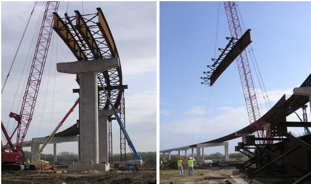
Figure 1.1 Early Stages of Curved I-Girder Bridge Construction
