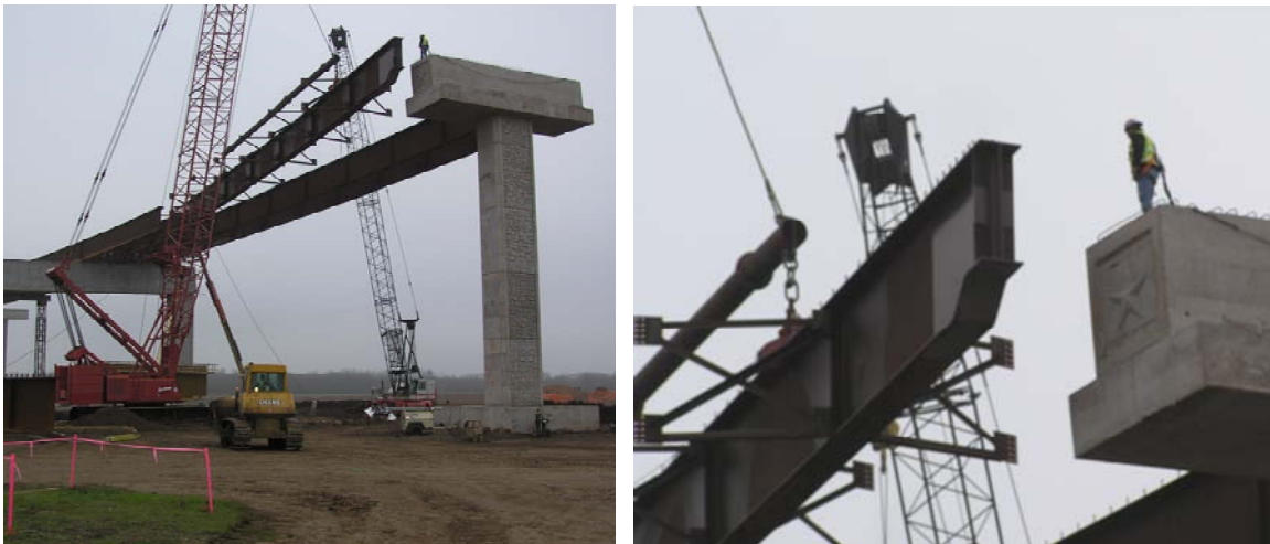
Figure 1.3 Single Crane I-Girder Erection
