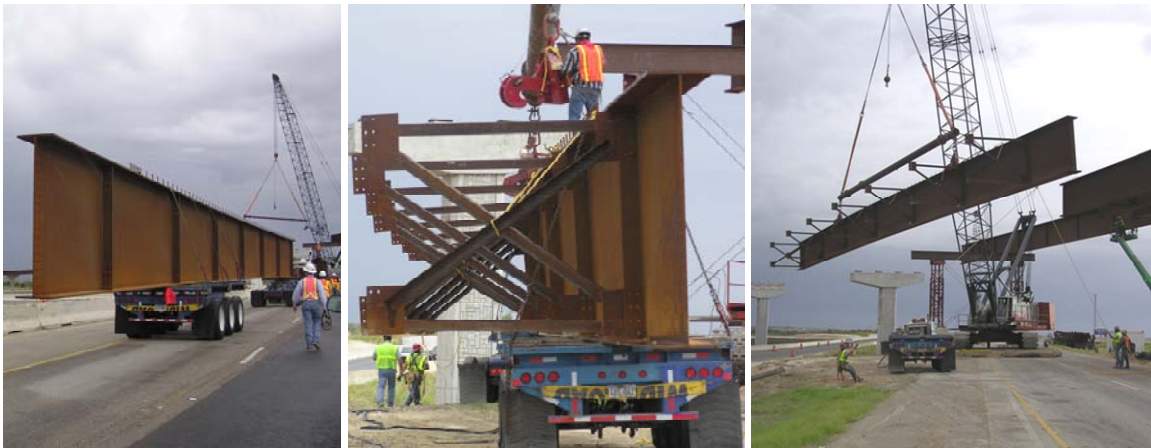
Figure 1.2 Girder Staged (a), Cross Frames Attached (b), Girder Erection (c)
